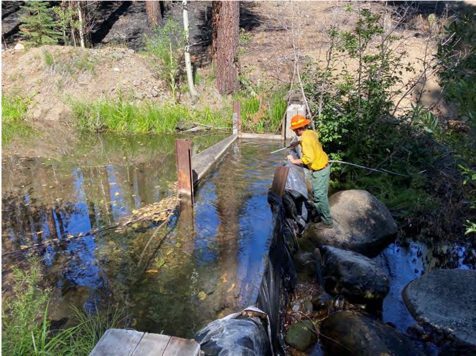
Photo 1: Pre-Tamarack Fire, the intake structure on Musser and Jarvis Creek consisted of a dam and a 14" pipe that extended into the upstream pond created by the dam. The pond measured about 30' long x 20' wide x 3' deep. Photo from BAER Report.
